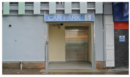
A new dedicated disabled lift was created on the ground floor which travels up specifically to the first floor only and is solely dedicated to Disabled users. For additional security the lift is locked at night and protected with roller shutters.
