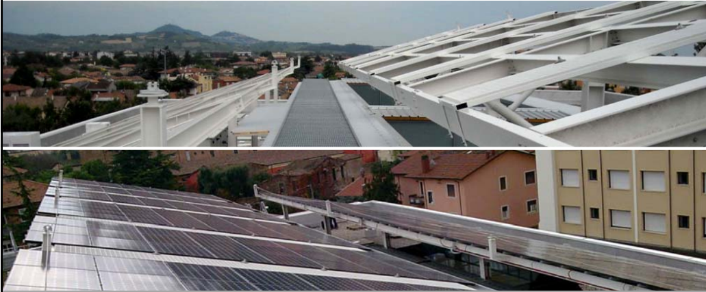
" IV Novembre" Car Park Project
