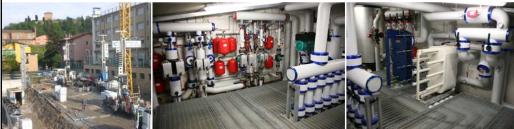
" IV Novembre" Car Park Project
