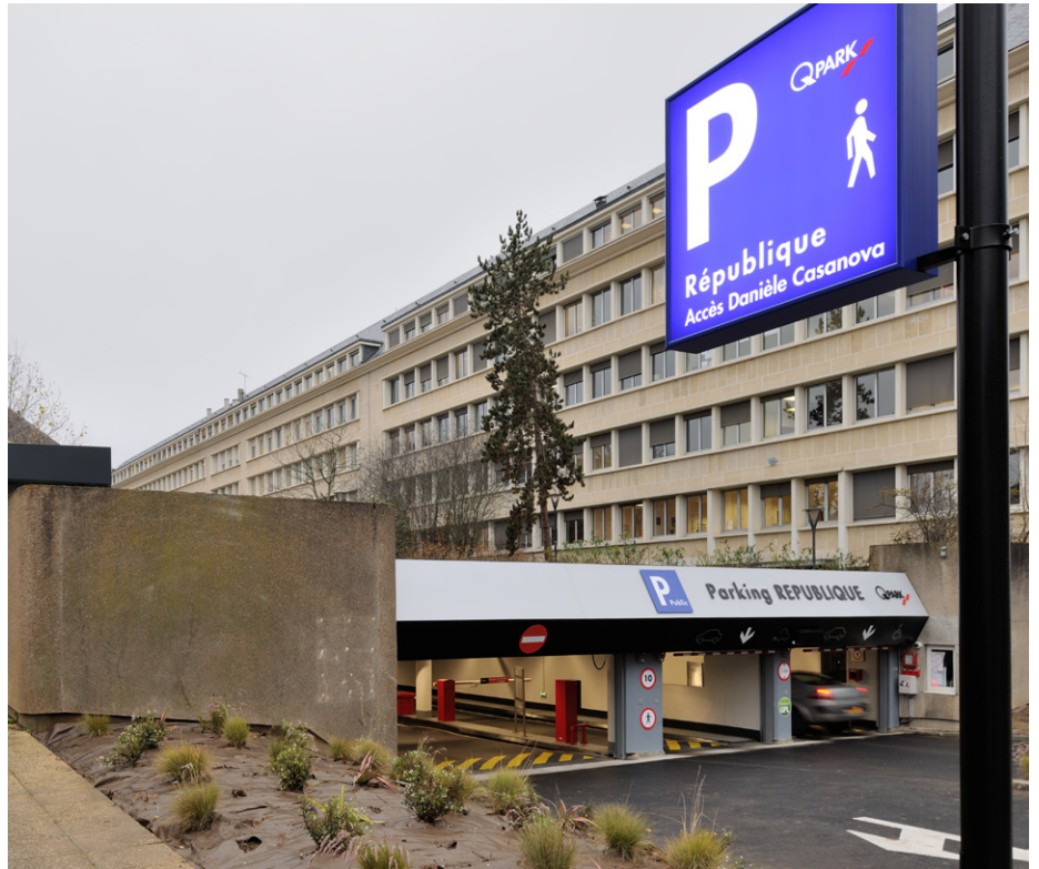
The Q-Park République car park in Chartres has 577 spaces.
