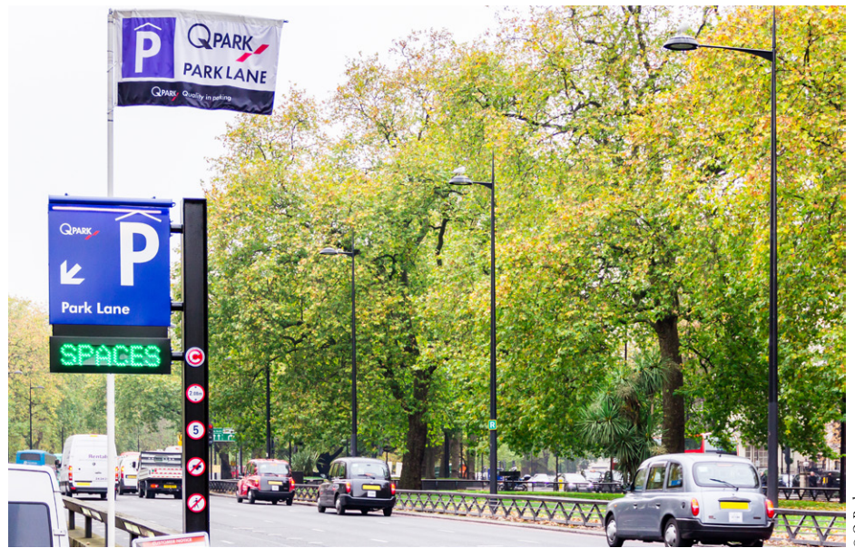
The new Park Lane Mobility Hub from Q-Park is located in the centre of London.
