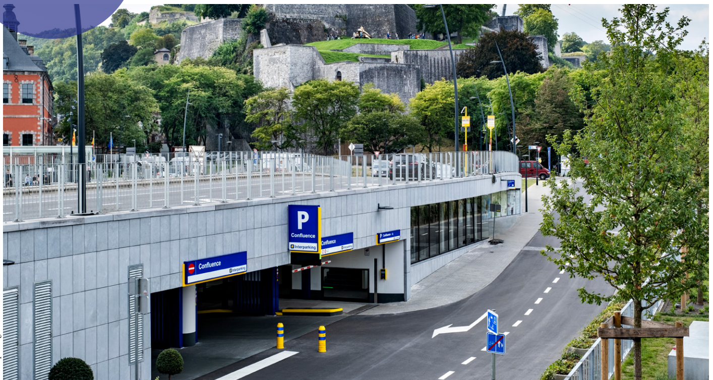
The new car park in Namur has 670 parking spaces and reaches up to twelve metres underground.
