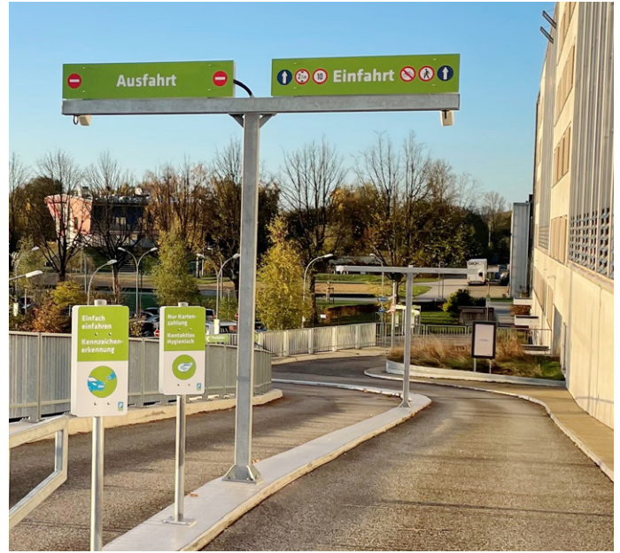
Entry and exit lane with two cameras each for number plate recognition from the front and the rear.
