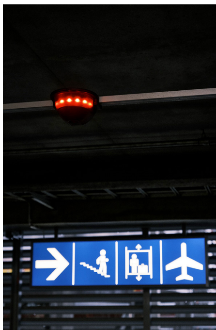
Green and red lights inform the customers about the availability of a parking space.
