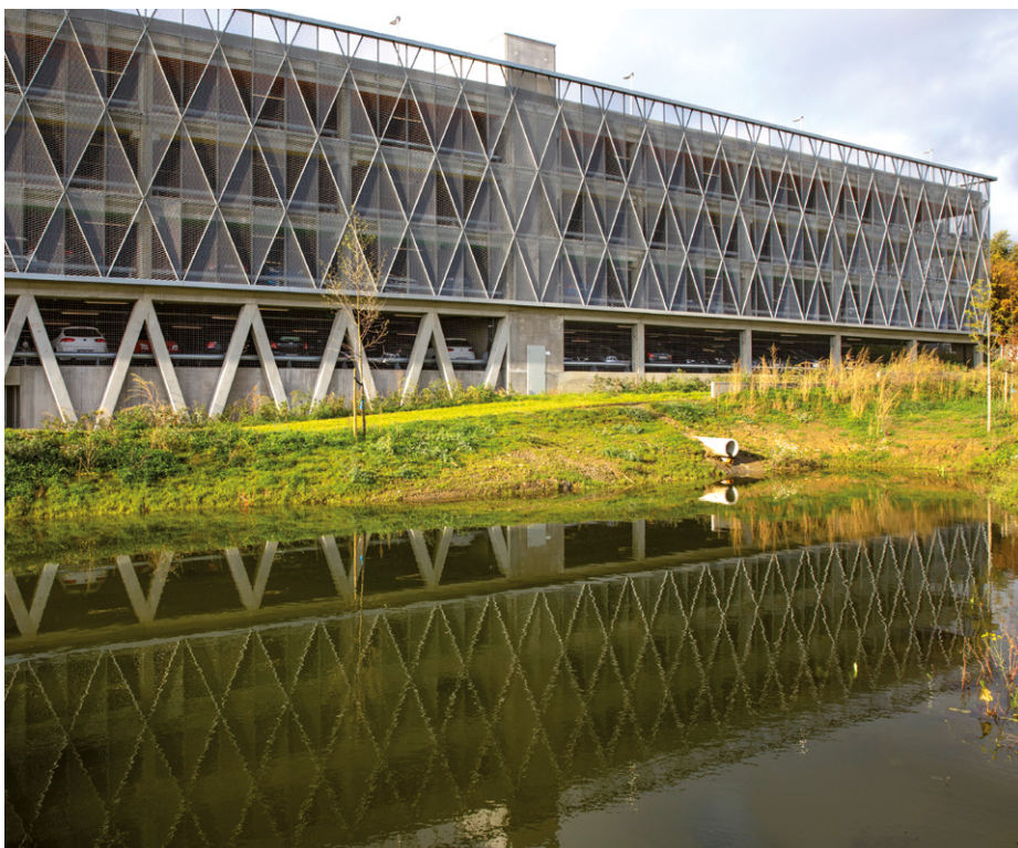
The new car park has a noise cancelling screen to reduce the sound from the ring road.
