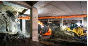
To keep the light in the car park during the construction and to be able to quickly start the surface development (including the building of a conference center), we used the "Stross hole" technique:
