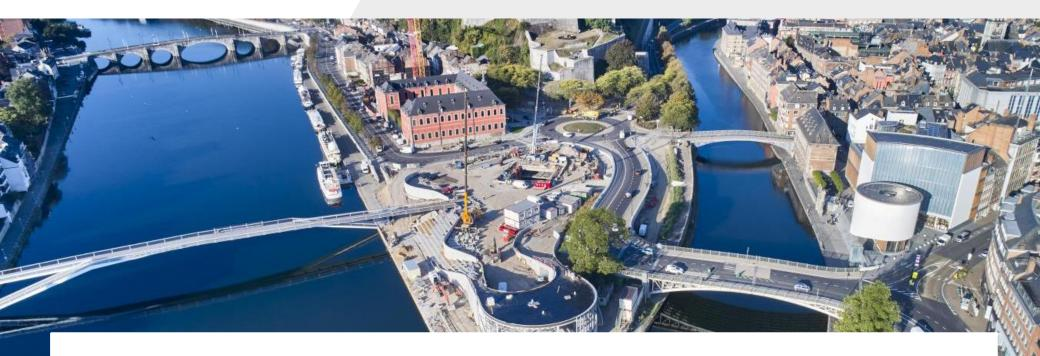
Given the location between two rivers and 9 meters below water level, this car park was designed as a floating boat, anchored in the rock. The weight of the structure was not sufficient to compensate for the water pressure. So, we placed no less than 400 anchors in the rock to ensure the stability of the structure. In addition, we had to provide several anti-flooding solutions.
