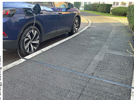
The innovative cross-pavement technology will allow cables to run safely beneath pavements, connecting homes directly to parked vehicles.
