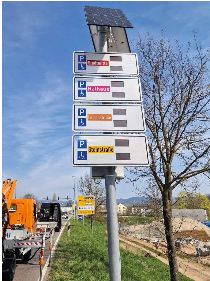
New parking guidance system in Emmendingen by MSR-Traffic
