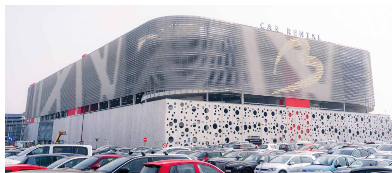
The new parking facility will serve as a central location for car hire services, within walking distance of the terminal.
