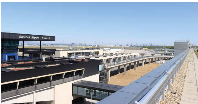
Up on the roof: the car park with a bridge connection to the new Terminal 3, with the Frankfurt skyline in the background.
