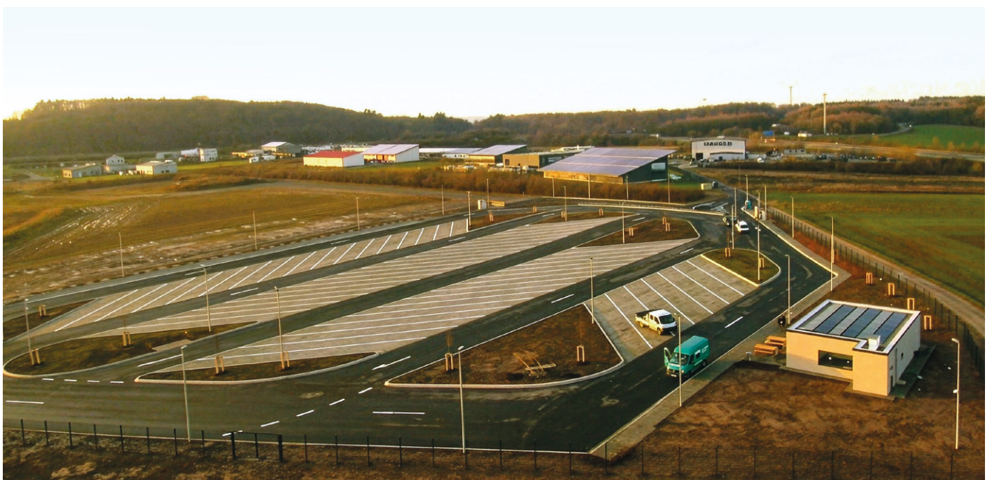
New secure truck parking area near Bitburg, equipped with barriers, video surveillance and digital parking management.
