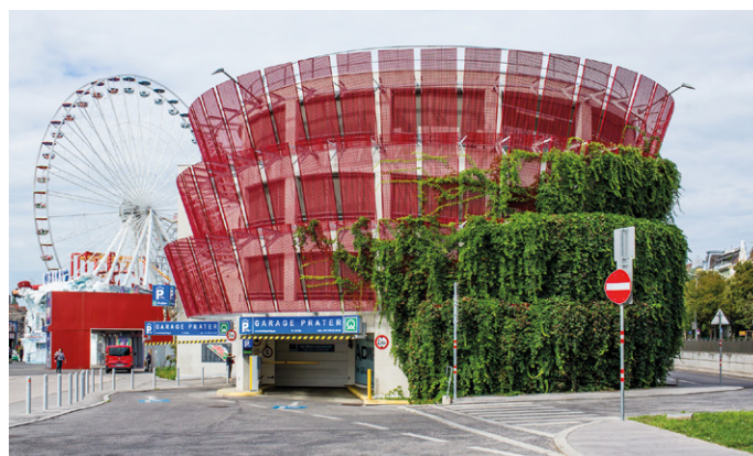
Sustainable and architecturally appealing: a multi-storey car park at Vienna's Prater with an innovative green façade
