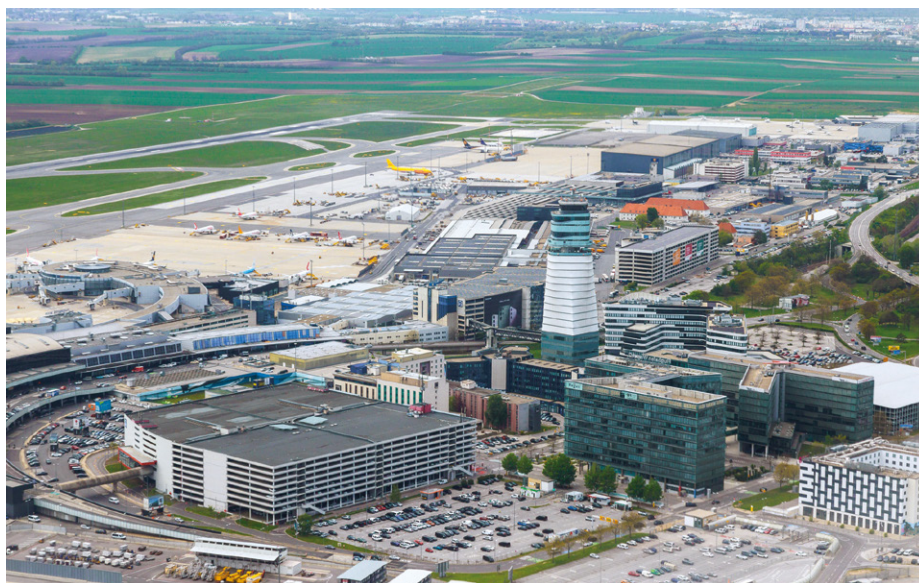
The “Turnaround-Center” is located in parking garage 4—in this picture the building at the front left—at Vienna Airport. Optimized processes save around 300 tons of CO 2 annually.
