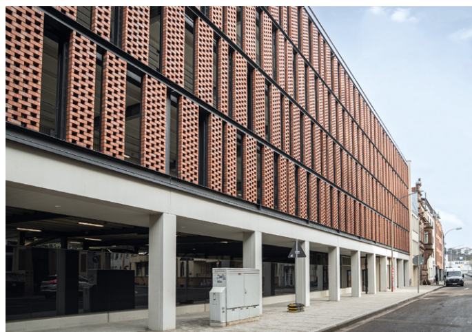
Architecturally striking: the unusual brick façade on the south side
