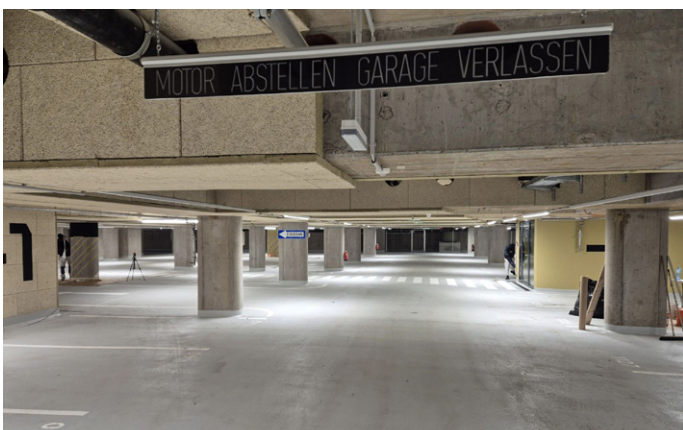
Warning sign for the CO alarm system
