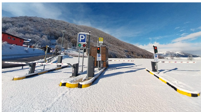
Entry and exit lane of Monte Pratello Cableway facilities
